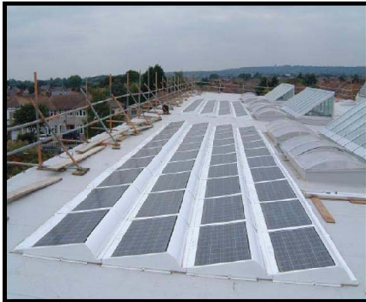
Figure 27: Actual Installation of Sharp NU Series panels with Solion SunMount® system
